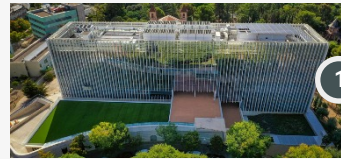
Barcelona Super Computing Centre: National supercomputing centre in Spain
