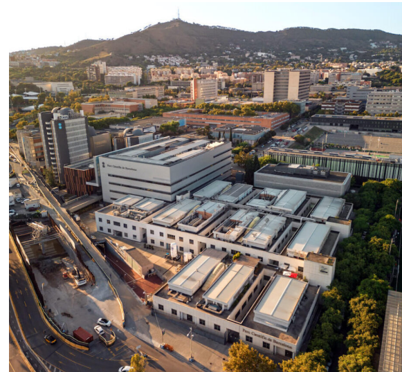
Science Park Area Hospital Clínic extension
